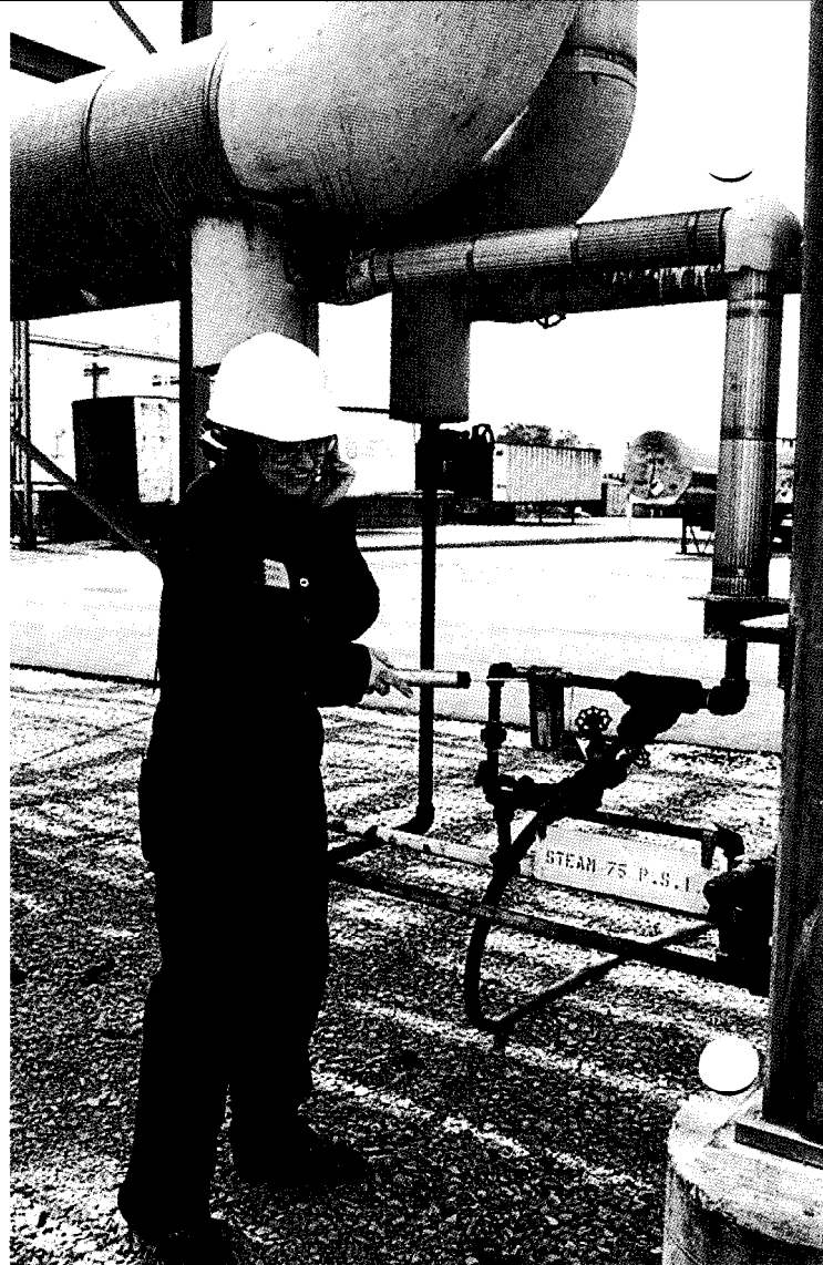
Fig. 2. A technician uses earphones to analyze the condition of this inverted bucket trap more precisely. Earphones should be used even if the sound test equipment is equipped with an optical gauge or dial to obtain a better analysis.
